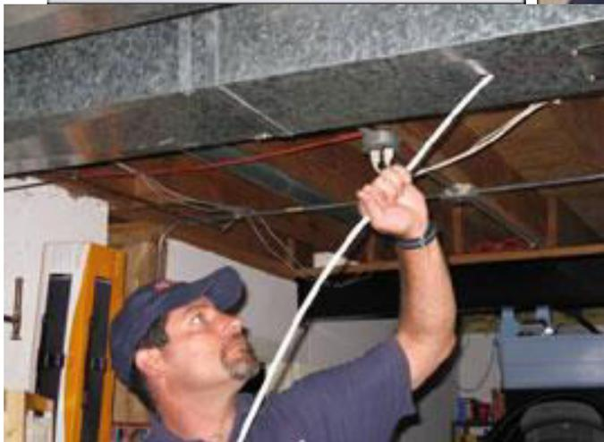
After mechanical brushing is complete, the Viper Rod system uses compressed air to mechanically agitate all surfaces of the ductwork, dislodging any remaining debris and pushing heavier contaminants toward the collection vacuum flow
