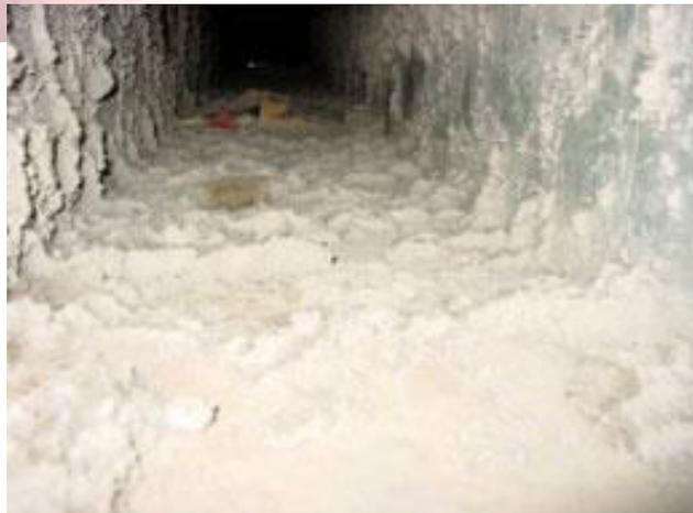
Properly cleaning HVAC systems requires removing the sources of contamination. Source removal begins with use of one or more agitation devices designed to loosen contaminants from the surfaces within the heating and air-conditioning system.
