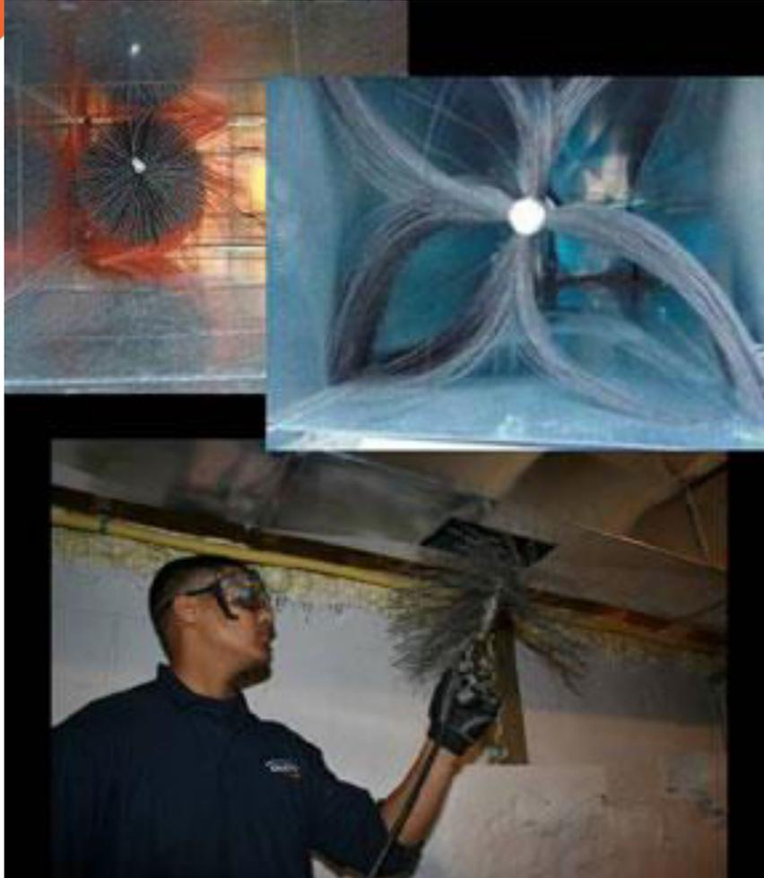
Brushes are selected based on the type of duct material. Silica Carbide brushes are the most aggressive method to agitate dirt and debris, but are only suitable for metal duct. Nylon brushes are selected for some metal ducts, and soft nylon brushes may be used on flexible mylar duct branches. Fiberglass lined ducts may require hand vacuuming.
