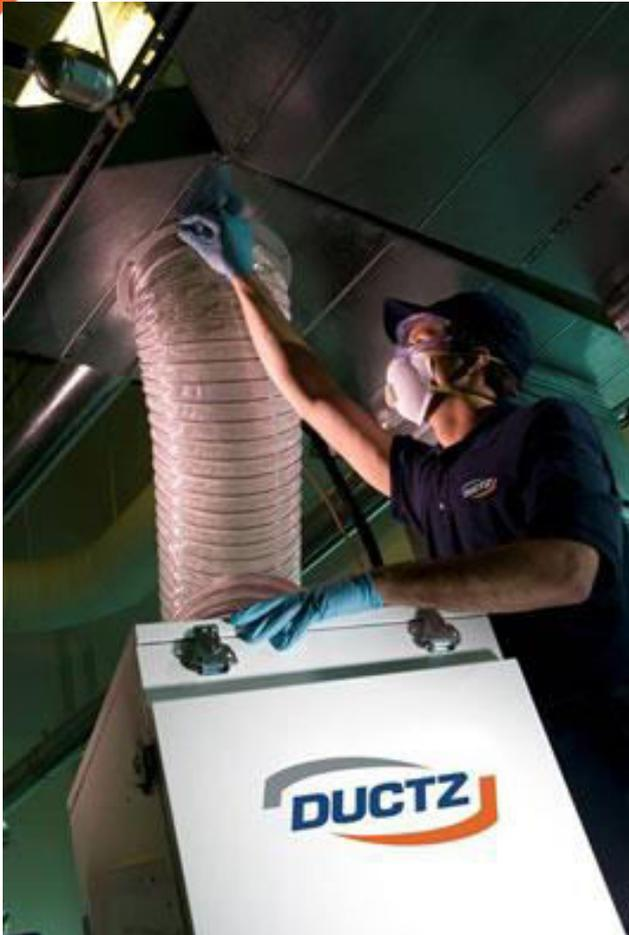
During cleaning, all register openings are sealed and the entire HVAC system is placed under continuous negative pressure (vacuum) to prevent the spread of contaminants.
