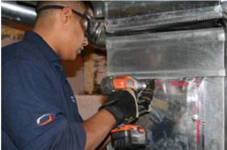
The Larger holes (where the negative air machine is attached to the duct) are sealed with sheet metal patches, zip screws and foil tape according to ACCA and SMACNA protocols.
