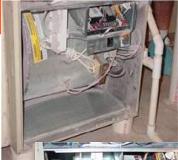
Remove the panel and use a HEPA filtered vacuum to remove debris from inside the unit. If debris on the blower is light and loose, we use HEPA filtered vacuum and compressed air to remove it (included in our basic service).
