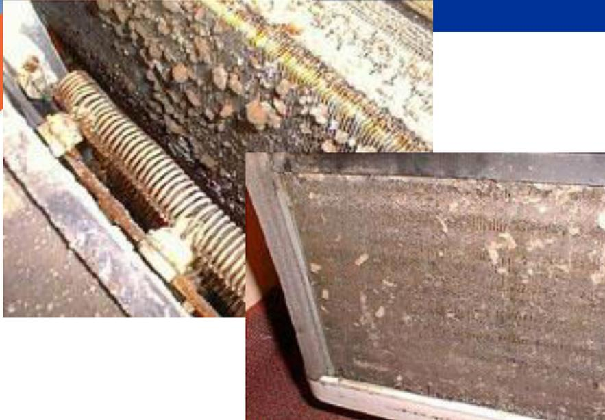
We Use a HEPA filtered vacuum to contact vacuum and compressed air to remove debris off of the coil when the debris is light and loose (often the case when good quality filtration is in place) – included in our basic service package
