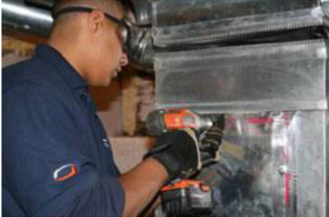
Access ports are cut into the supply and return sides of the system so that the HEPA filtered negative air collection unit may be connected. These access holes are 8" to 12" in diameter and will be properly sealed upon completion.
