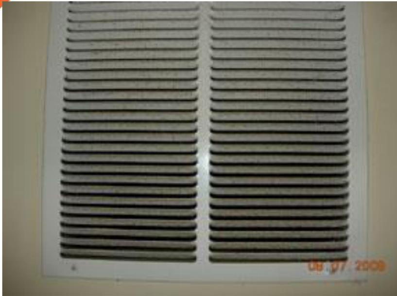
Registers and diffusers must be removed to properly clean the branch lines
